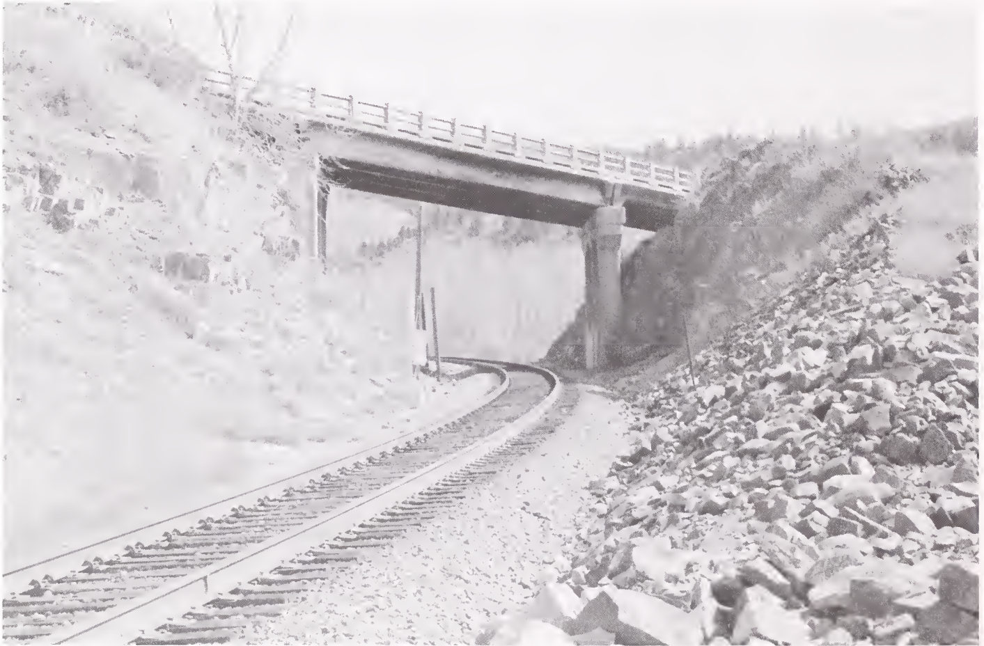
Northern Pacific Overpass Bridge near Garrison in Powell County.
